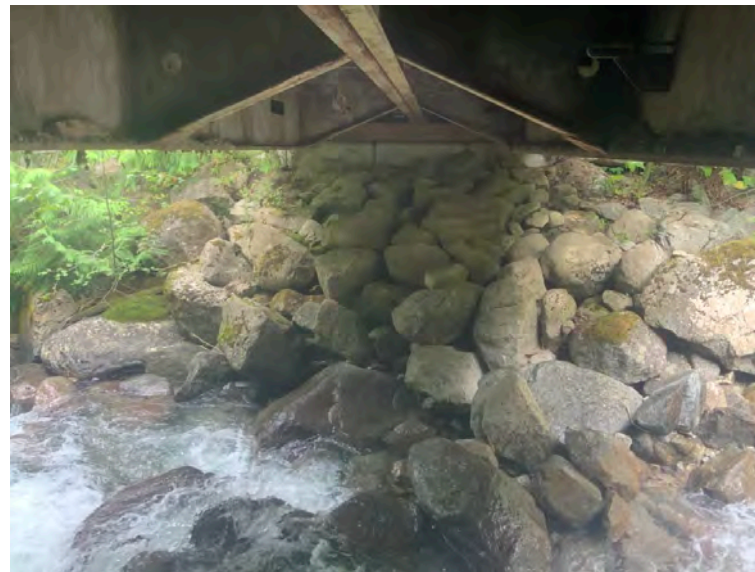
Right Bank Abutment when facing downstream
