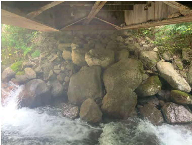
Left Bank Abutment when facing downstream
