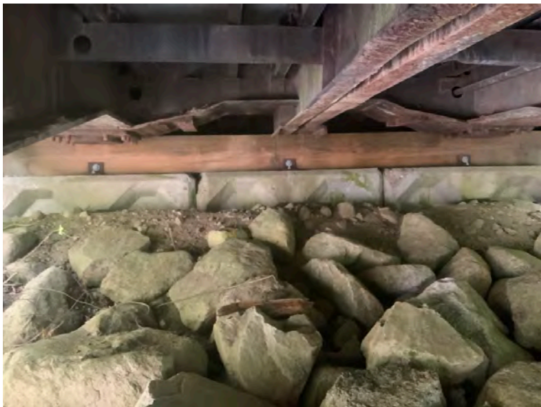
Left Bank Abutment when facing downstream
