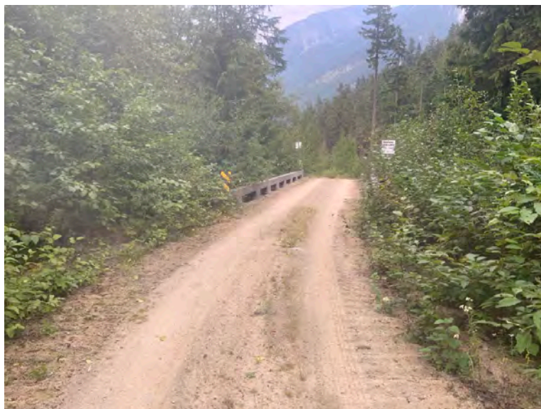
Approach from Left Bank when facing downstream
