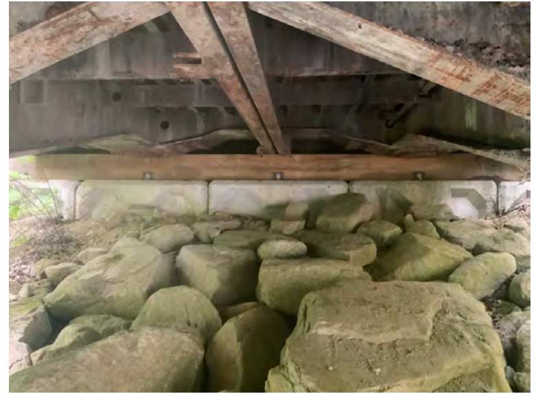
Right Bank Abutment when facing downstream
